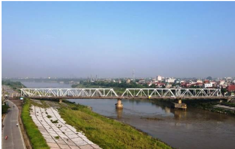
Figure 12: Low vertical clearance of Duong Bridge makes it difficult for large barges to pass through
